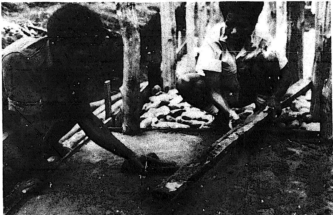
Plate 5. Concrete floor surface. A wood float finish is the best surface to have.
