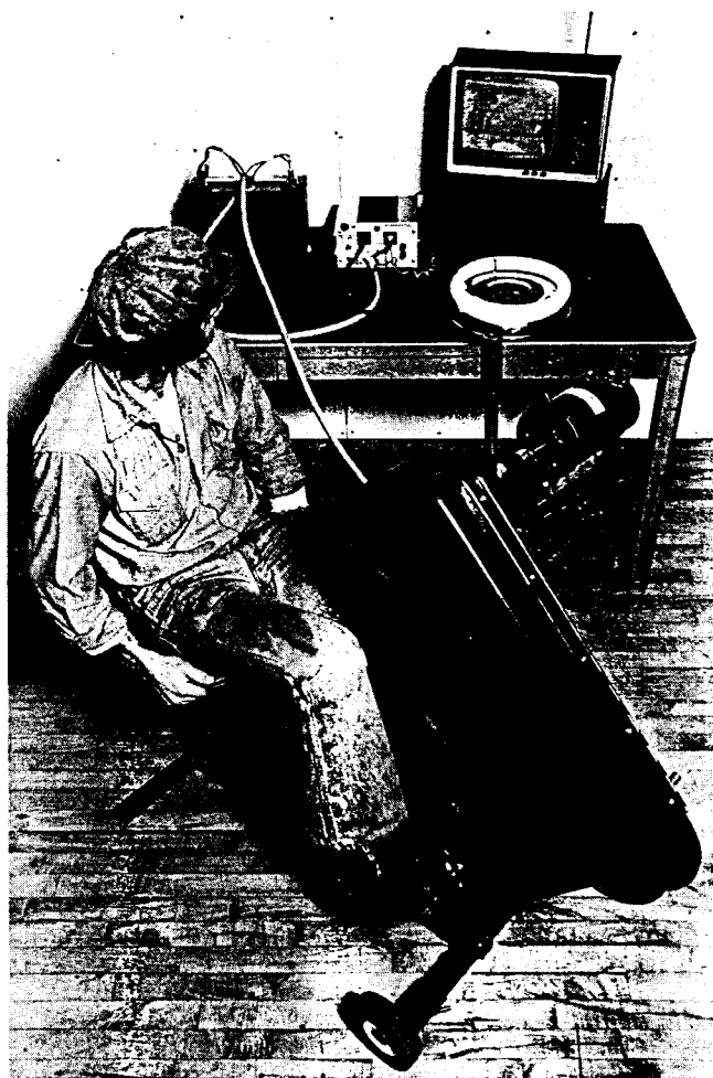
Figure 3-14 Generating electricity with the Energy Cycle
