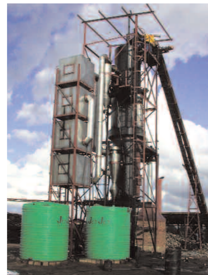
Figure 2: RWC's Slow Pyrolysis facility
