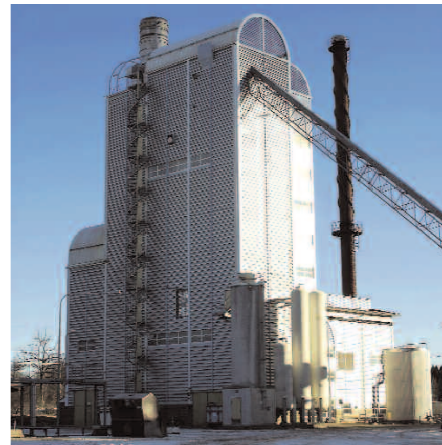
Figure 1: The Värnamo Plant, Sweden.
