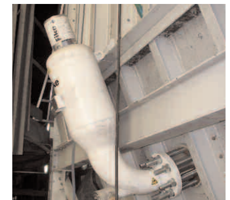
Figure 4 a & b: Anti-explosion bottles for protecting the fuel bins and pipes conveying air and wood dust mixtures.
