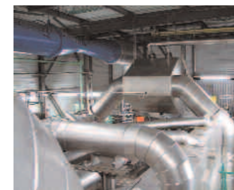
Figure 3: View of the boiler top
