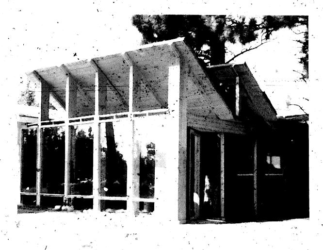
The roof is supported by 4 "x-12" hollow box beams that span twenty feet. There is a six we drop from west to east for drainage. The entire solarium has a light open feeling like a high roofed cathedral. with pine trees growing through the roof.
