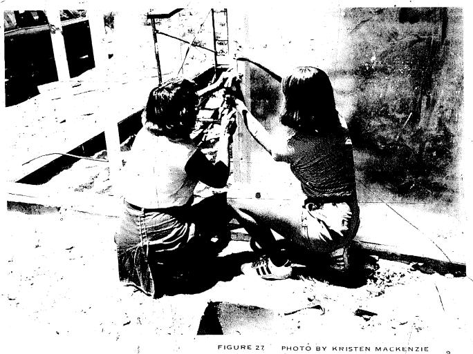
The irregular shaped plinels in the corners of the east and west wall are sized by cutting a rectangular piece to fit the length of the frame. Hold the piece up to the panel and mark the shape with a chalk line. Save the scraps for other irregular shapes and yents.
