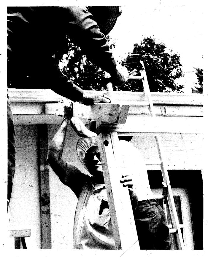
The next step is to cut and place the lower plates on the east and west walls (No. 3, Figure 23). Bolt the plates down. To connect the frame walls of the greenhouse to the home, a stud is securely "tied-in" to the home wall. It should fit snugly from the bottom plate to directly under the rafter plate (No. 4).
