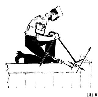
Figure 1-12.-Using a wrecking bar.
