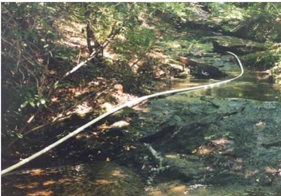
Figure 8. A PVC drive pipe placed in a stream bed. Galvanized steel was not an option due to the bed topography and geometry. The hydraulic ram pump worked well, but each bend allowed a tiny portion of the shock wave to dissipate. A straight, galvanized steel pipe would have captured a larger shock wave and provided more pressure. Photo credit: W. Bryan Smith, Clemson University.
