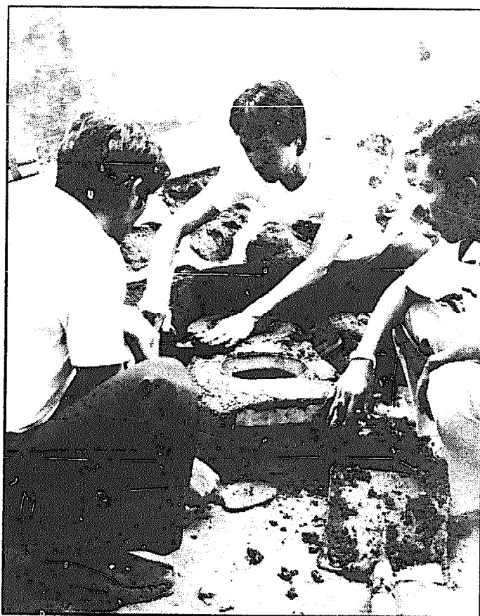
Plastering on the protective insulating liner.
