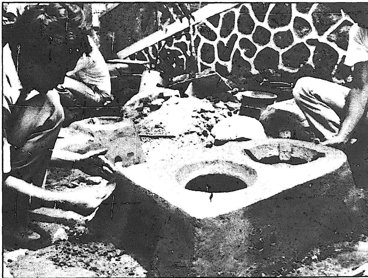
Village cadre studying "Lowon" style stove construction.
