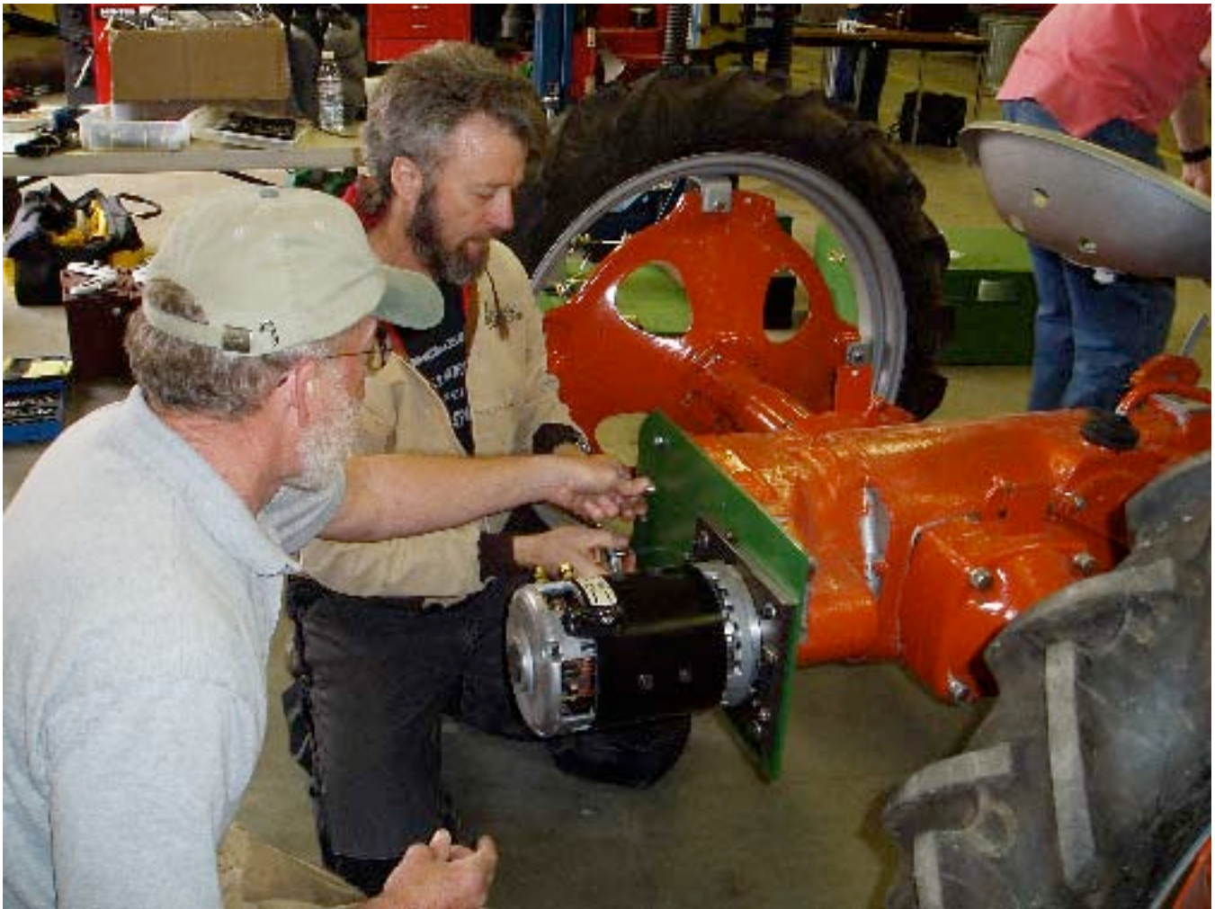
Motor plate installation.
