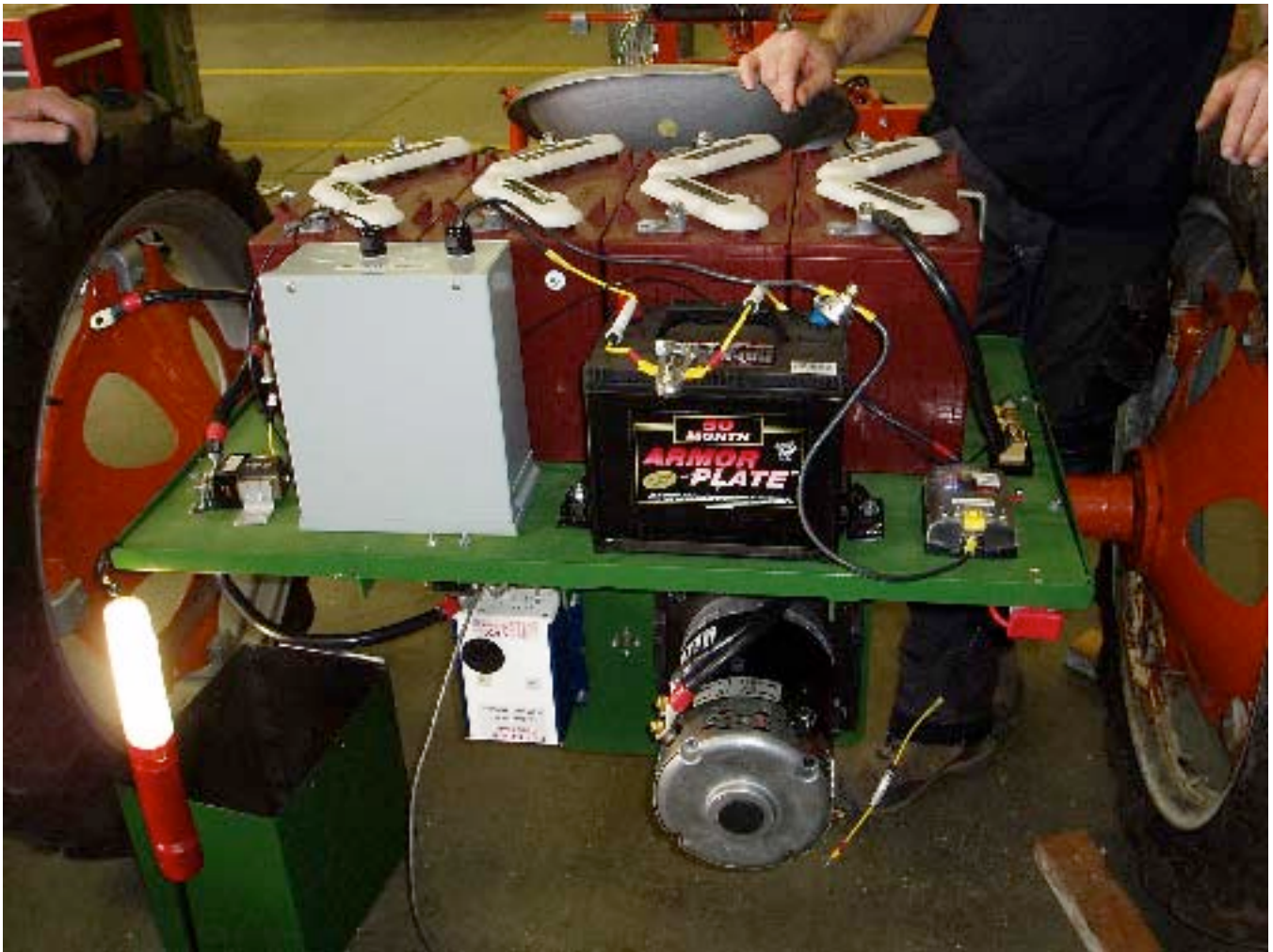
Battery rack and battery bank installation.
