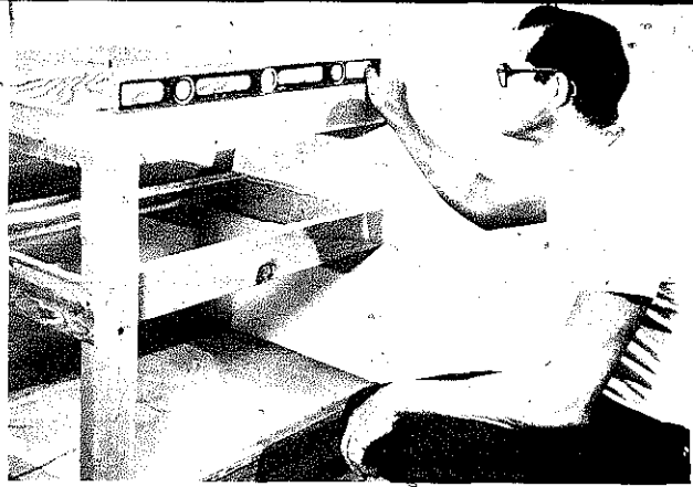
Be sure the bench frame is level. Check frequently as you proceed after you have installed the 2 x 4s on the walls. Work with a level - not a square.
