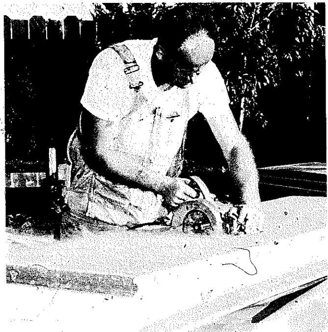
On soft materials like this roof-deck insulation, you can make a maximum cut on one surface and then snap the material to break uncut section. If appearance of the cut is important, then, of course, you must cut from both sides.
