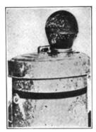
FIG. 129. — An effective combination garbage can and fly trap. (After Hodge.)
