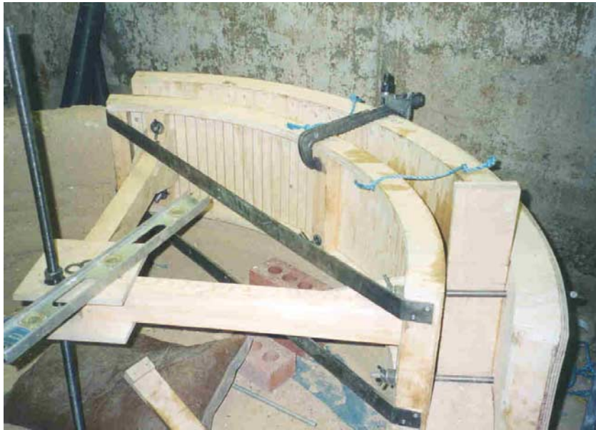
Figure 7.3 – Shuttering manufactured in the UK
