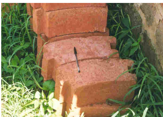
(Figure 6.3 – Curved blocks after curing)
