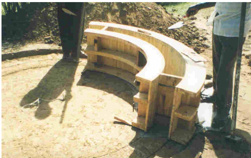
Figure 7.4 Shuttering manufactured in Uganda
