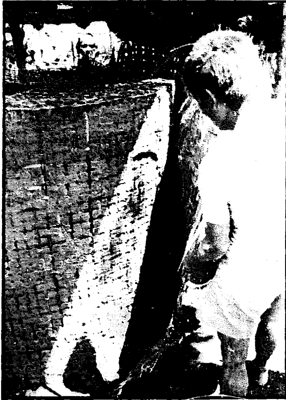
Left: removing the supportive mats Right: plastering the outer wall
