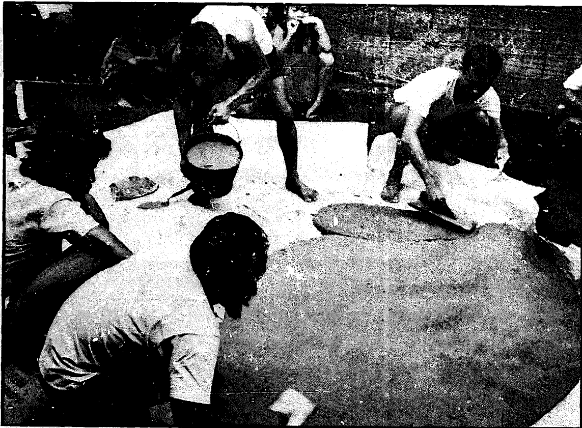
Plastering the foundation: be sure soil does not pollute the plaster
