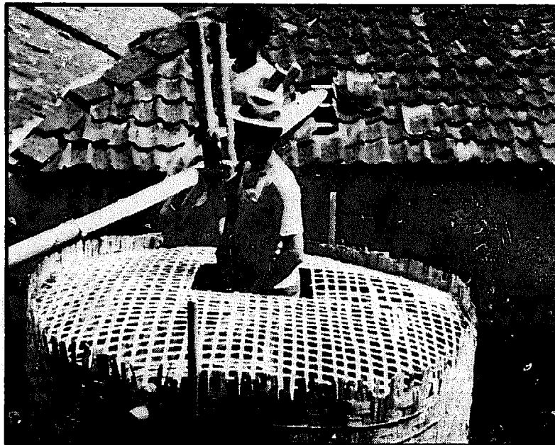
scaffolding for easy entry and exit
