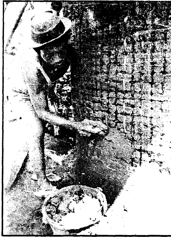
Left: removing the supportive mats Right: plastering the outer wall
