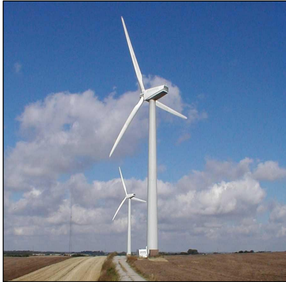
Figure B-1 The Norwin 46-ASR-600 kW turbines Ørsted 2 (in front) and Ørsted 1 used in the measuring program. The wagon containing the measuring equipment is seen besides Ørsted 2, and the measuring mast is seen to the left of the road.
