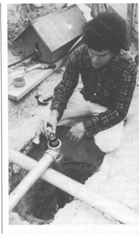
Figure 5.3. Seating the bottom check value in an open top cylinder. Make certain that paper or cardboard pro tectors are removed from the ball value.
