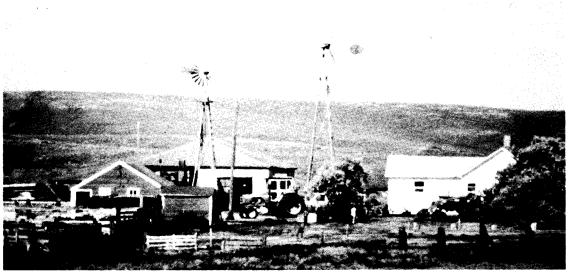
**Figure 2.3.** A low-solidity, high-speed wind rotor for electricity generation (right) and a high-solidity, slower-speed wind rotor for mechanical applications (left).
