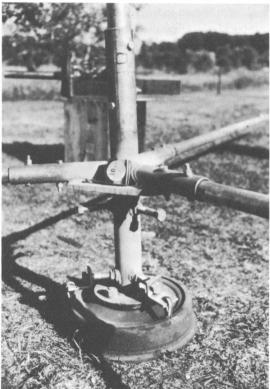
Figure 4.21. Guy cable attachments on the hub bolts.
