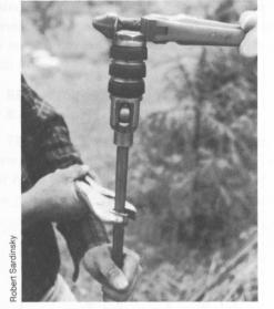
Figure 5.5. Attaching the plunger to the pump rod.
