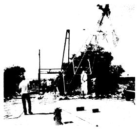
Figure 5.11. Hoisting the windmill and tower at the same time.
