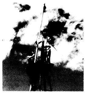
Figure 5.15. A gin pole in place on the tower.
