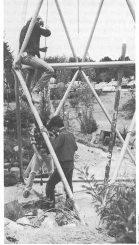
Figure 5.7. Station an elevated person above the well when lowering the pump rod.
