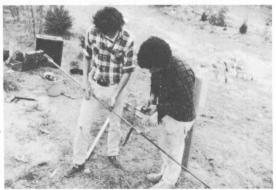
Figure 5.6. When attaching sections of pump rod, be sure to avoid bending the rod.
