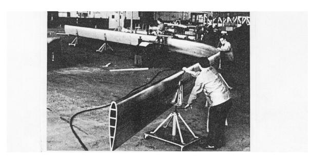
Figure 6: Extruded aluminum blade of 17-m Darrieus during fabrication. (Courtesy of Aluminum Company of America.)
